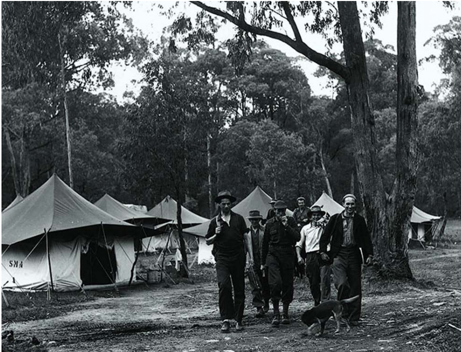
A surveying team leaving the Indi Camp in 1951 (photo from https://www.snowyhydro.com.au/about/history/ ).
